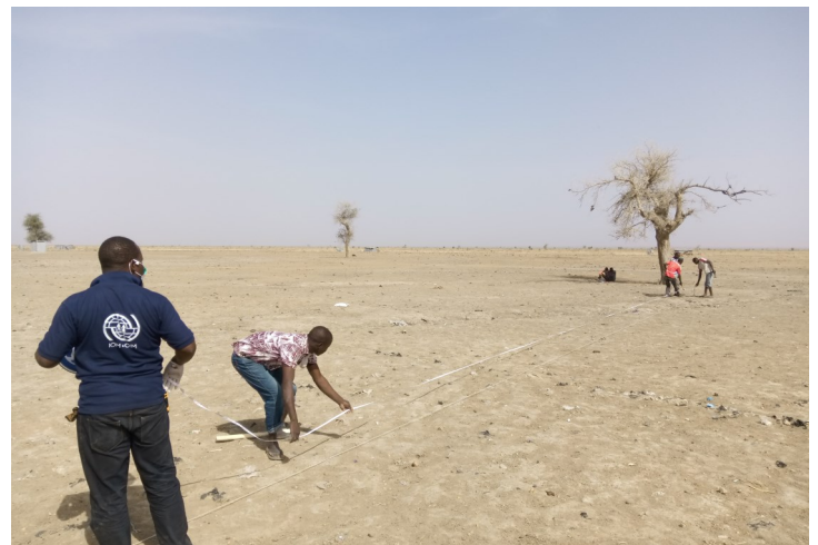
Construction of self-quarantine shelter in Pulka, Borno State. Photo: © IOM 2020
