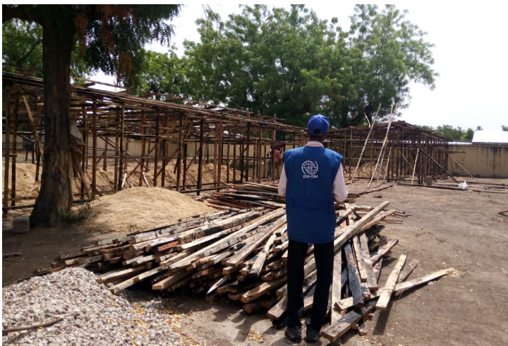
Construction of self-quarantine shelters in Bama, Borno State. Photo: © IOM 2020
