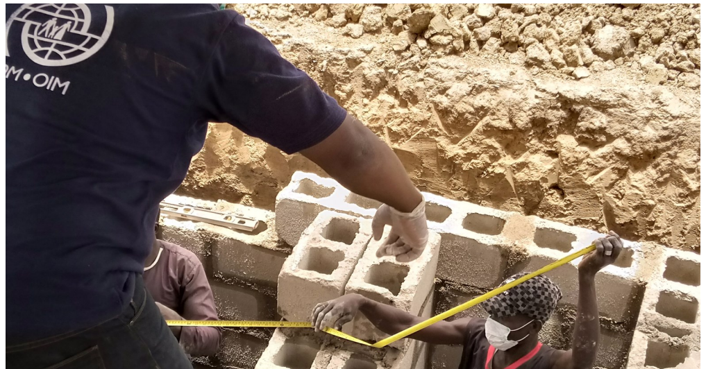
Construction of self-quarantine shelter in Borno State. Photo: © IOM 2020
